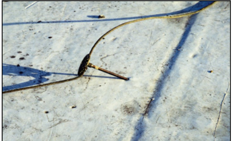
Damage to roof membrane from loose and wind-blown lightning rod. Source: Everest Loss Control Files
